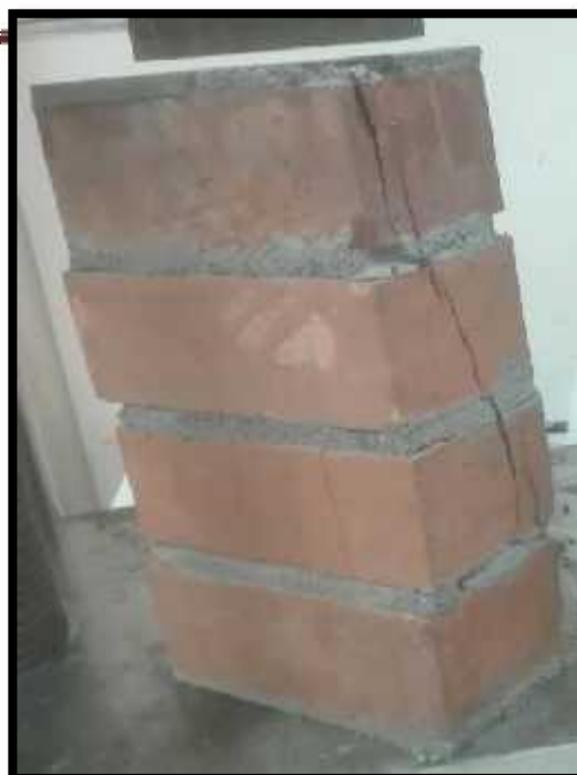
Figura 37. Fisura vertical vista frontal – Semi industrial.
