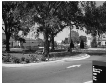
Fig. 3.2—Pervious concrete pavement used within the drip line of tree.
