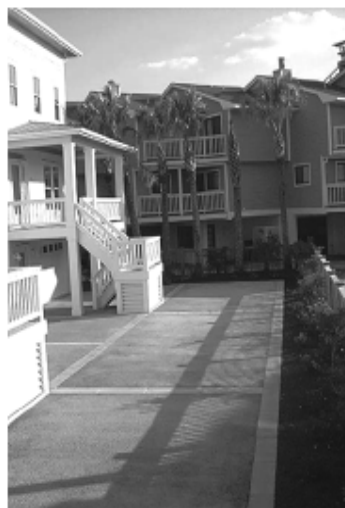
Fig. 3.1—Parking lot built with pervious concrete pavement.
