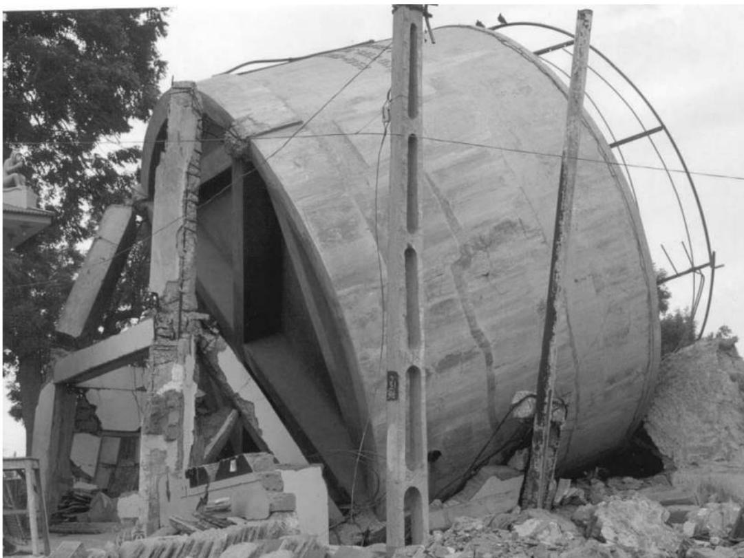
*Nota.* Reproducida de Severe damage to similar staging required that the water tank be pulled down in Bhachau., de Drugesh Rai, 2003, Performance of elevated tanks in Mw 7.7 Bhuj earthquake of January 26th, 2001.
