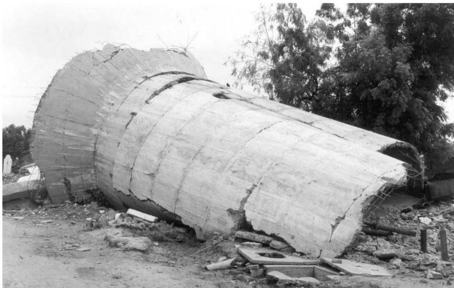
*Nota.* Reproducida de Collapsed 265 kL water tank in Chobari village about 20 km from the epicenter, de Drugesh Rai, 2003, Performance of elevated tanks in Mw 7.7 Bhuj earthquake of January 26th, 2001.
